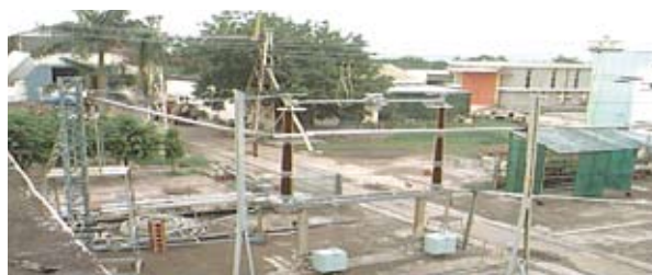
420kV Horizontal Central Break Isolator with Flexible Conductor
